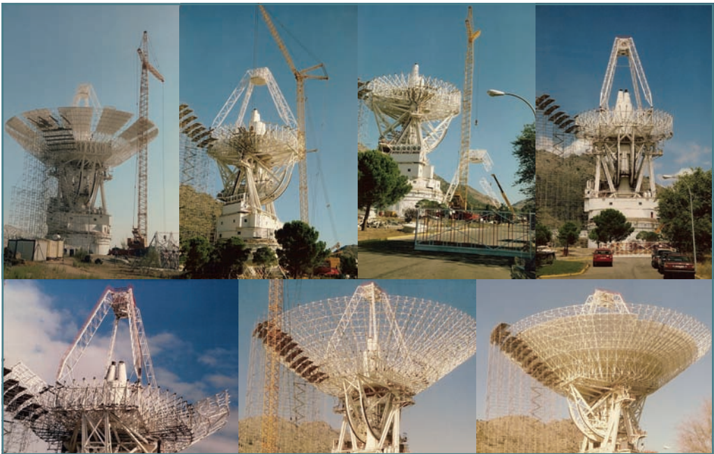
Sequence extending to 70 m with a very high scaffolding and rotations of the antenna. ■
