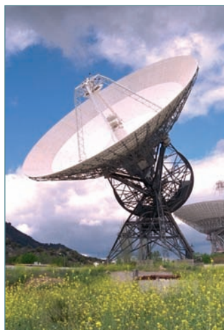
Photographs of the antenna DSS 61 in the process of modification, and already converted to 34 m. The enlarged part of the reflector, the X band cone, and the concrete blocks in the feet can be seen. ■
