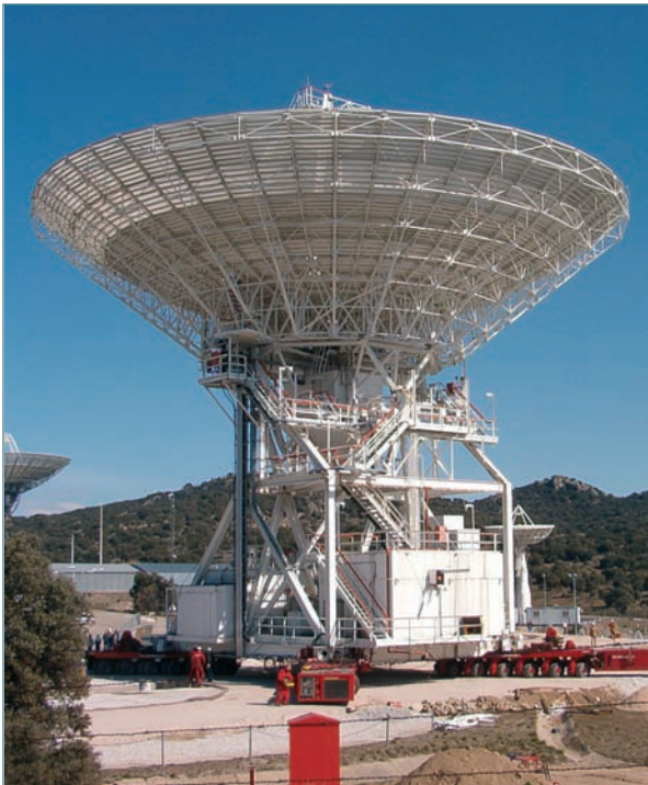
Photos with detail of the "tractors" and the antenna being relocated. ■
