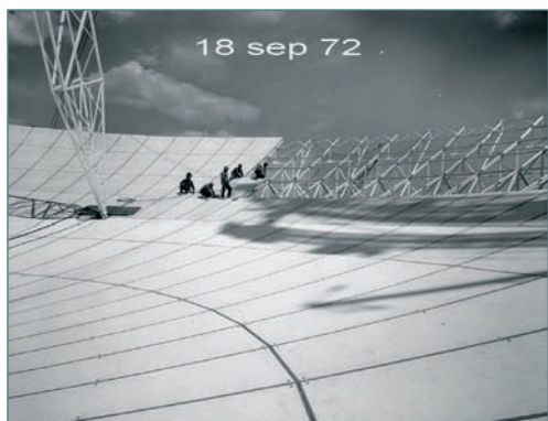
Photographic sequence of the construction of the large antenna. ■
