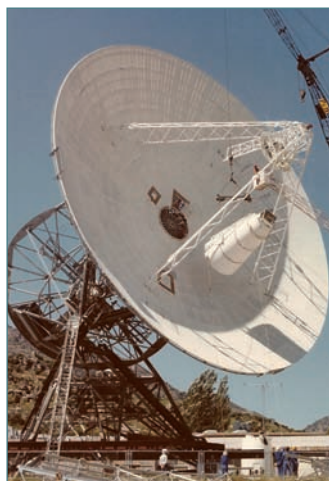
Photographs of the antenna DSS 61 in the process of modification, and already converted to 34 m. The enlarged part of the reflector, the X band cone, and the concrete blocks in the feet can be seen. ■
