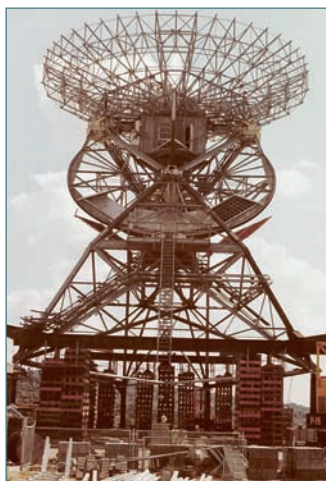
Photographs of the antenna DSS 61 in the process of modification, and already converted to 34 m. The enlarged part of the reflector, the X band cone, and the concrete blocks in the feet can be seen. ■
