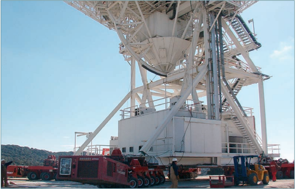
Photos with detail of the "tractors" and the antenna being relocated. ■
