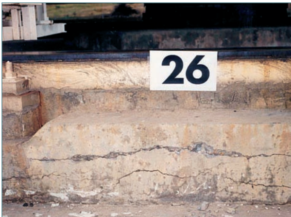
Aspect of the pedestal cracks. ■
